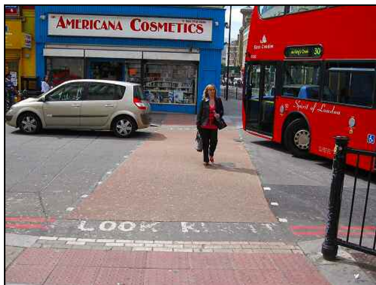
Plate 4.12: Lack of controls at crossing C18 across King's Cross Bridge placing pedestrians in danger of turning traffic
