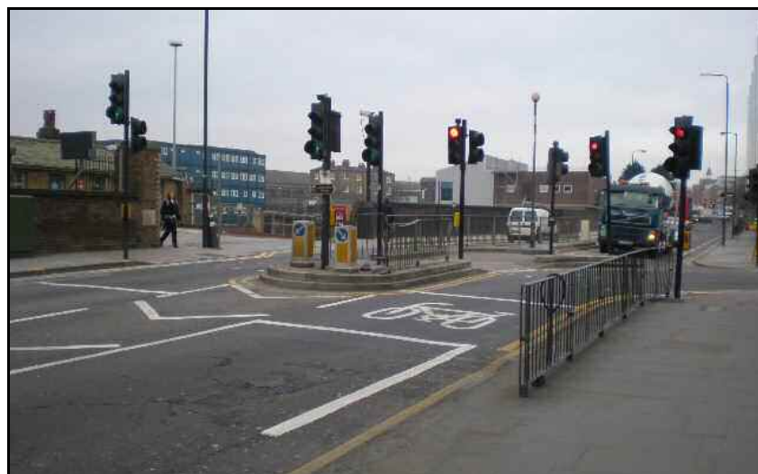
Plate 4.19: Poor alignment of crossing arms at C52
